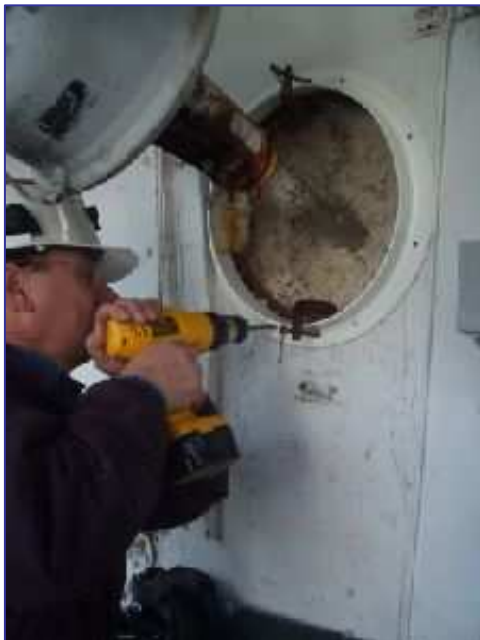
Figure 120.2 Installation of CB Casing Bulkhead Ring
