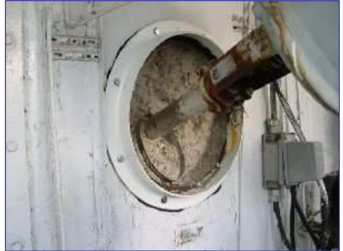
Figure 120.3 Completed Installation of CB Casing Bulkhead Ring
