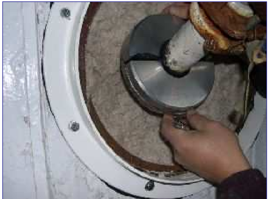
Figure 120.4 Installation of Stem Collar
