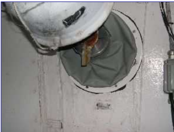
Figure 120.6 CB Boot Installation Complete
