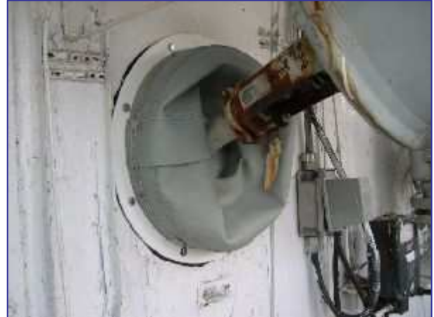
Figure 120.7 CB Boot Installation Complete
